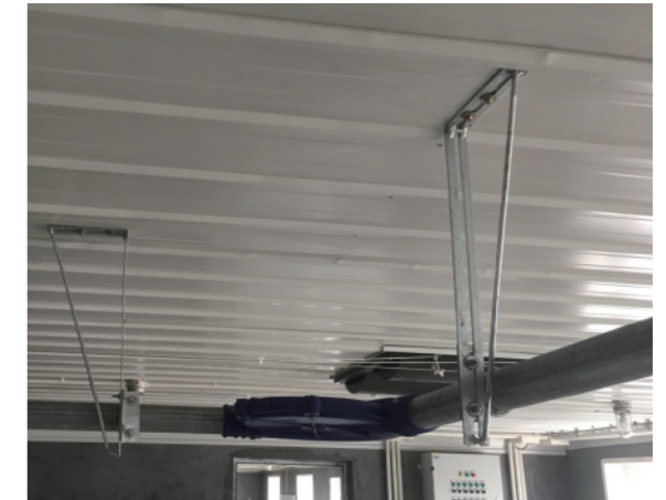
转角轮安装 Installation of Corner Wheel
